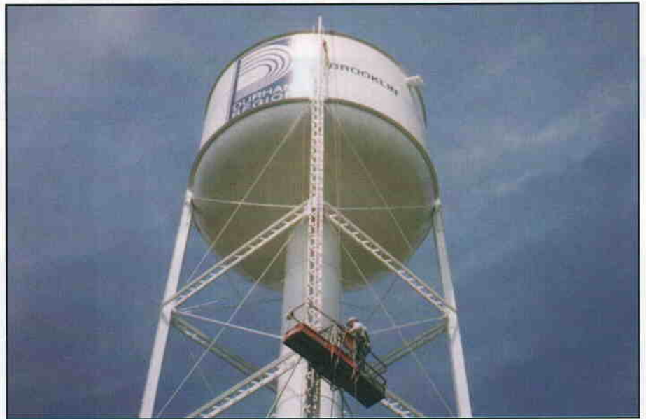
Engineered Coatings Ltd. worked with Madison Chemical to repair the Brooklin Water Tower, and now it looks like new
