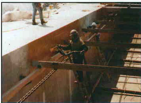
Wastewater clarifier in Hamilton Ontario coated with Madison's Flexcel II TX
