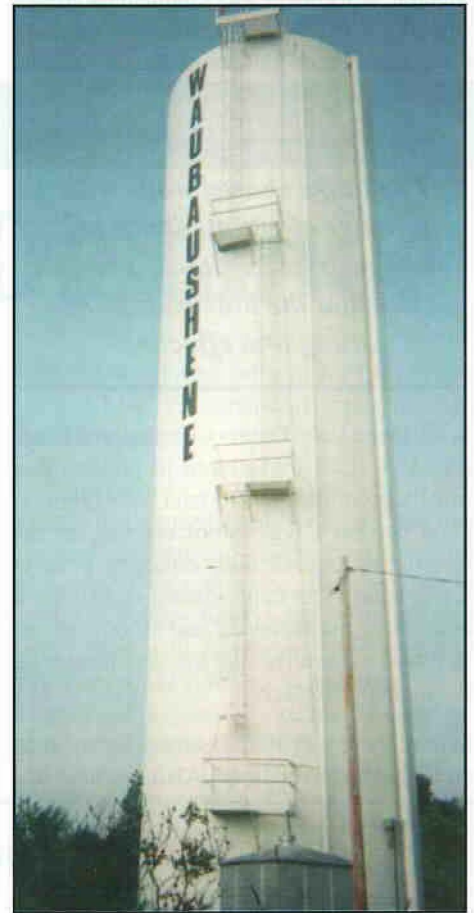
Waubauskene potable water storage tank
